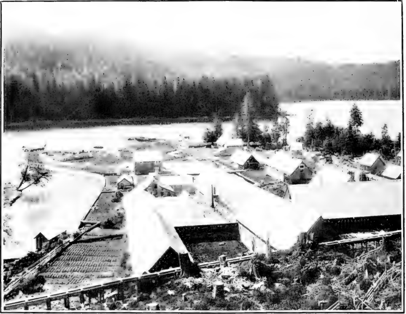
FIG. 45.—ALASKA PACKERS ASSOCIATION FORTMANN HATCHERY, NAHA STREAM, ALASKA
